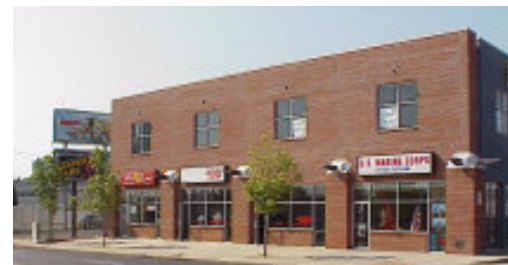
710 Marietta Street / retail, office & warehouse
