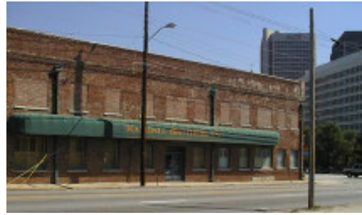
655 Marietta Street / Randall Brothers Building Materials
